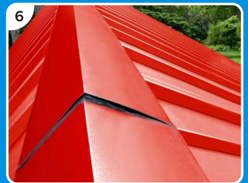
6 Fix loose or damaged flashings immediately
