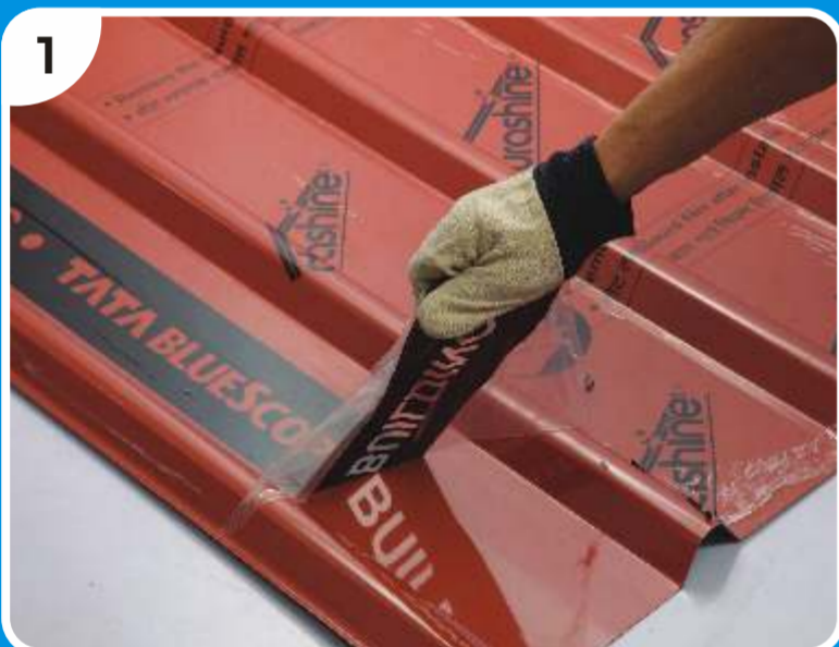
1 Remove guardfilm immediately after installation
