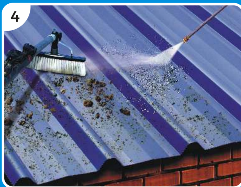
4 Clean dirt in valleys with water and soft bristled brush regularly
