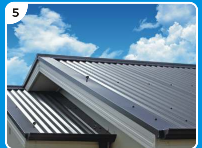
5 Check regularly for loosened nails, rivets & screws
