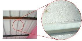
Condensation is the natural formation of water droplets on the bottom side of any installed metal roofing sheet. It may occur when there is a difference in temperature between the air in the building and the sheet itself, causing the water vapour (moisture) in the air to condense on the inside of the sheet. It is a natural phenomenon and hence no claims will be entertained in this regard.
